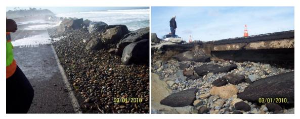
**Figure 2.** Flooding and undermining of Highway 101 in the study area during a March 2010 event. Courtesy of City of Encinitas.
